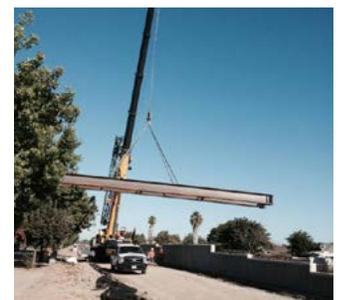
250-ton crane lifting the 44,000-lb, 78-ft Valley Green pedestrian bridge into place
