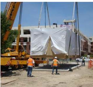
Setting the TPSS into place on the foundation pad
